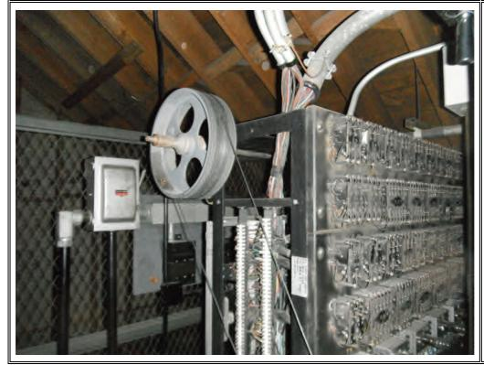
Traction elevator with points and contact controls in the attic space, maintenance provided by Southern Elevator.
