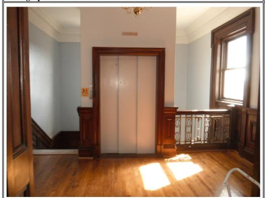
Elevator stop at third floor. Cab rated for 1500lbs and has current certification.
