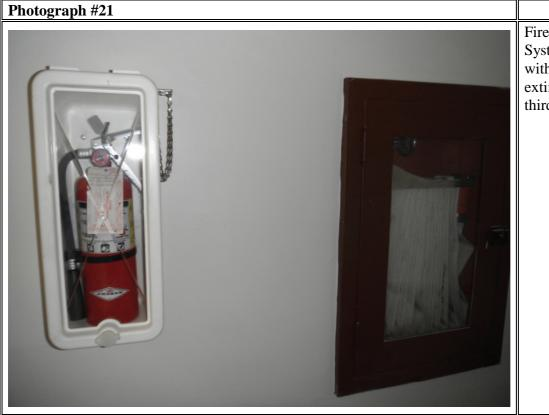
Fire Life and Safety System stand pipe with fire hose and fire extinguisher on the third floor
