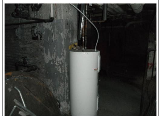
52-gallon electric water heater in basement services restrooms and break room. Photo Date: February 23 & 24, 2017 Page 9 of 16
