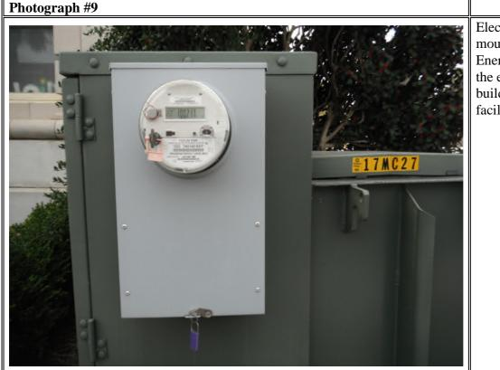
Electrical pad mounted Progress Energy transformer at the east side of the building servicing facility
