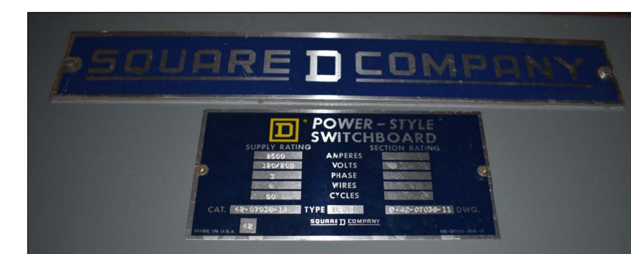
4 PHOTO: SWITCHBOARD NAMEPLATE E-1 NOT TO SCALE
