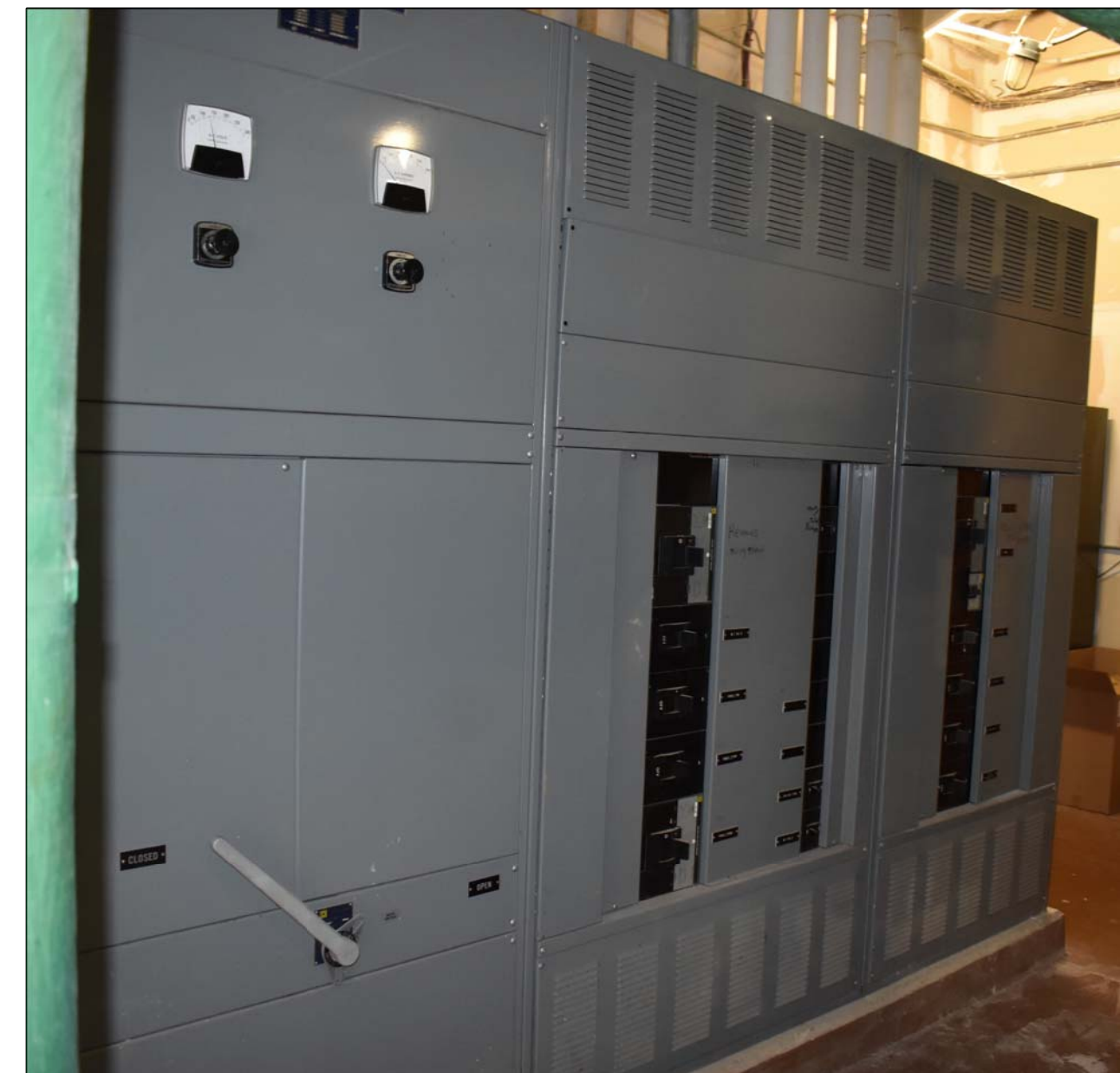
3 PHOTO: EXISTING SWITCHBOARD E-1 NOT TO SCALE
